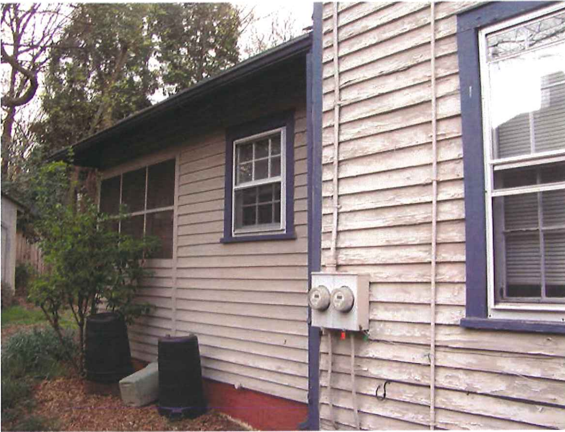
View of partial south facade, rear of residence
