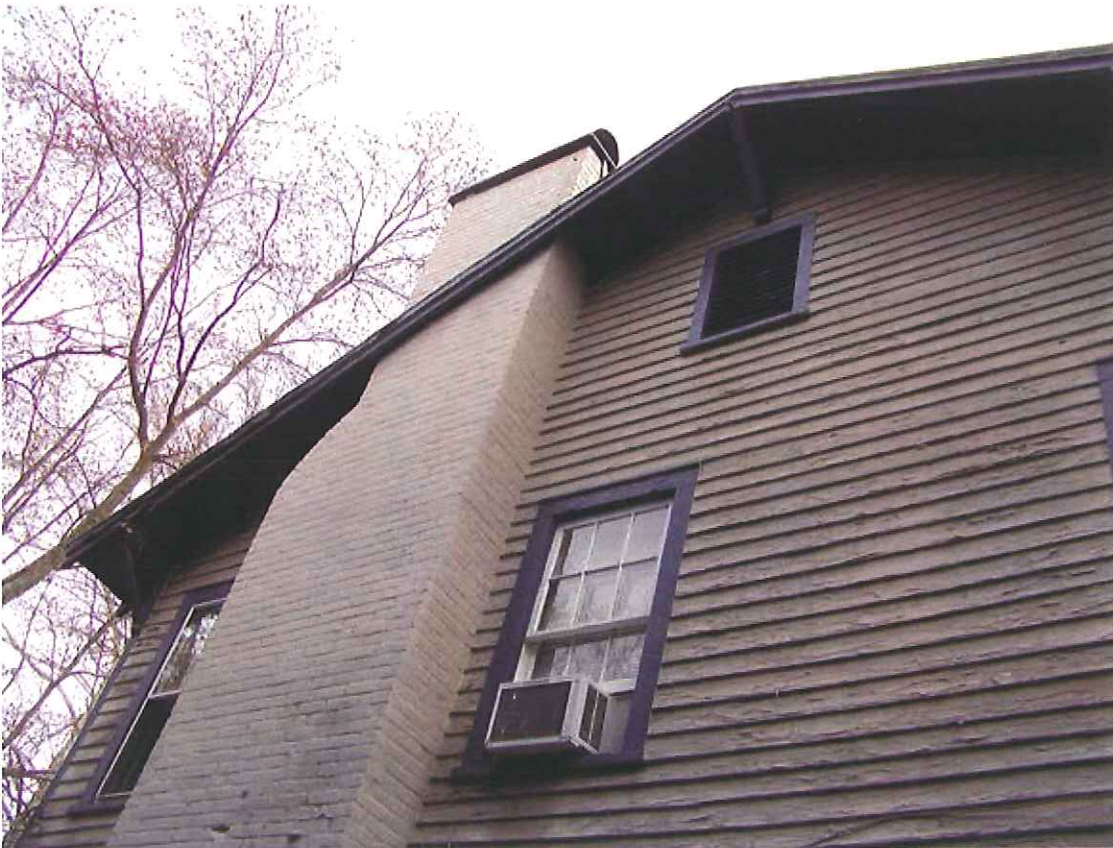
North facade, partial view
