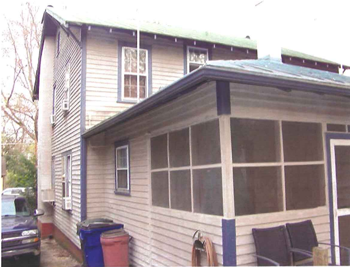
View of northwest corner of residence showing existing screen porch
