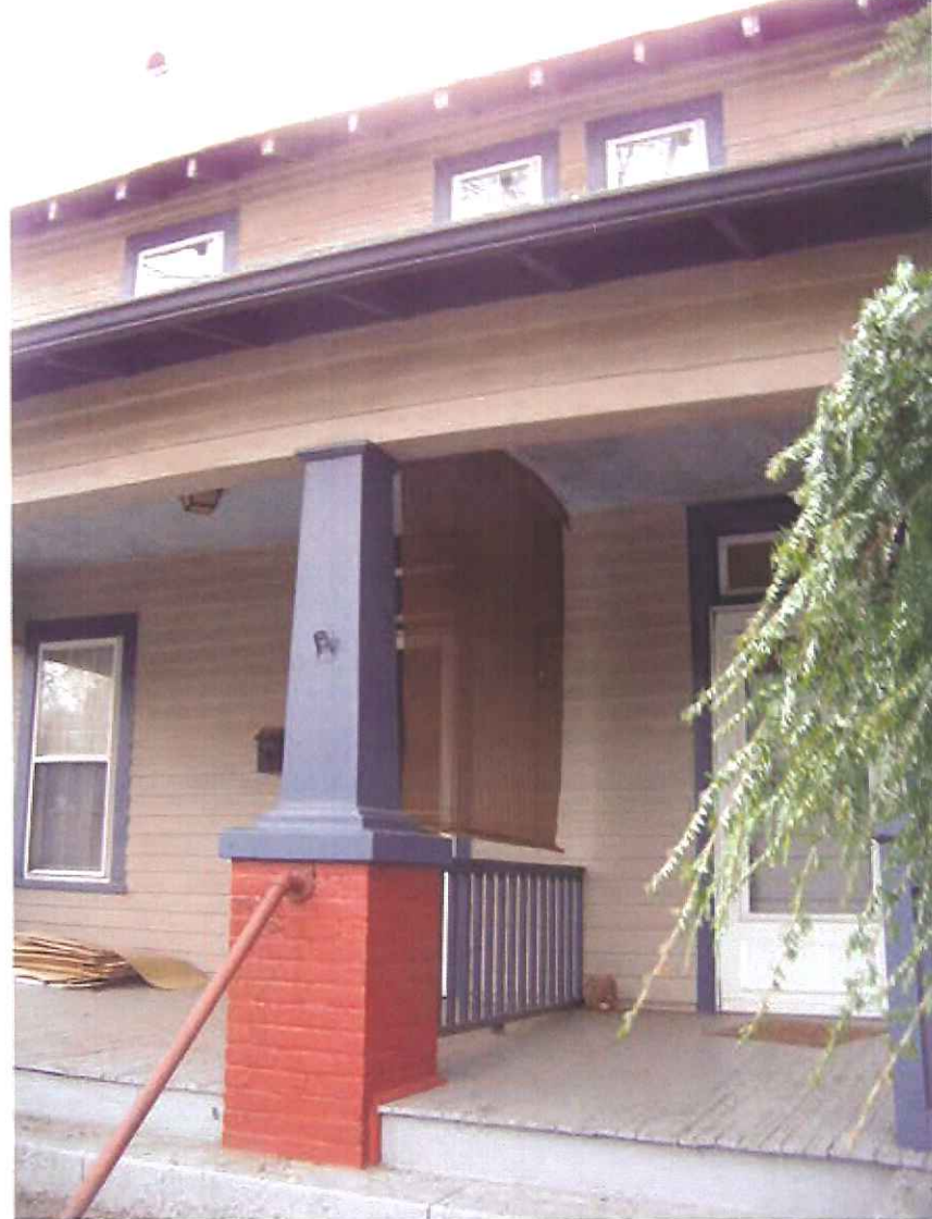
View of front porch showing central rail
