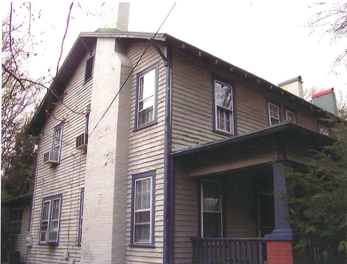
View of partial south facade
