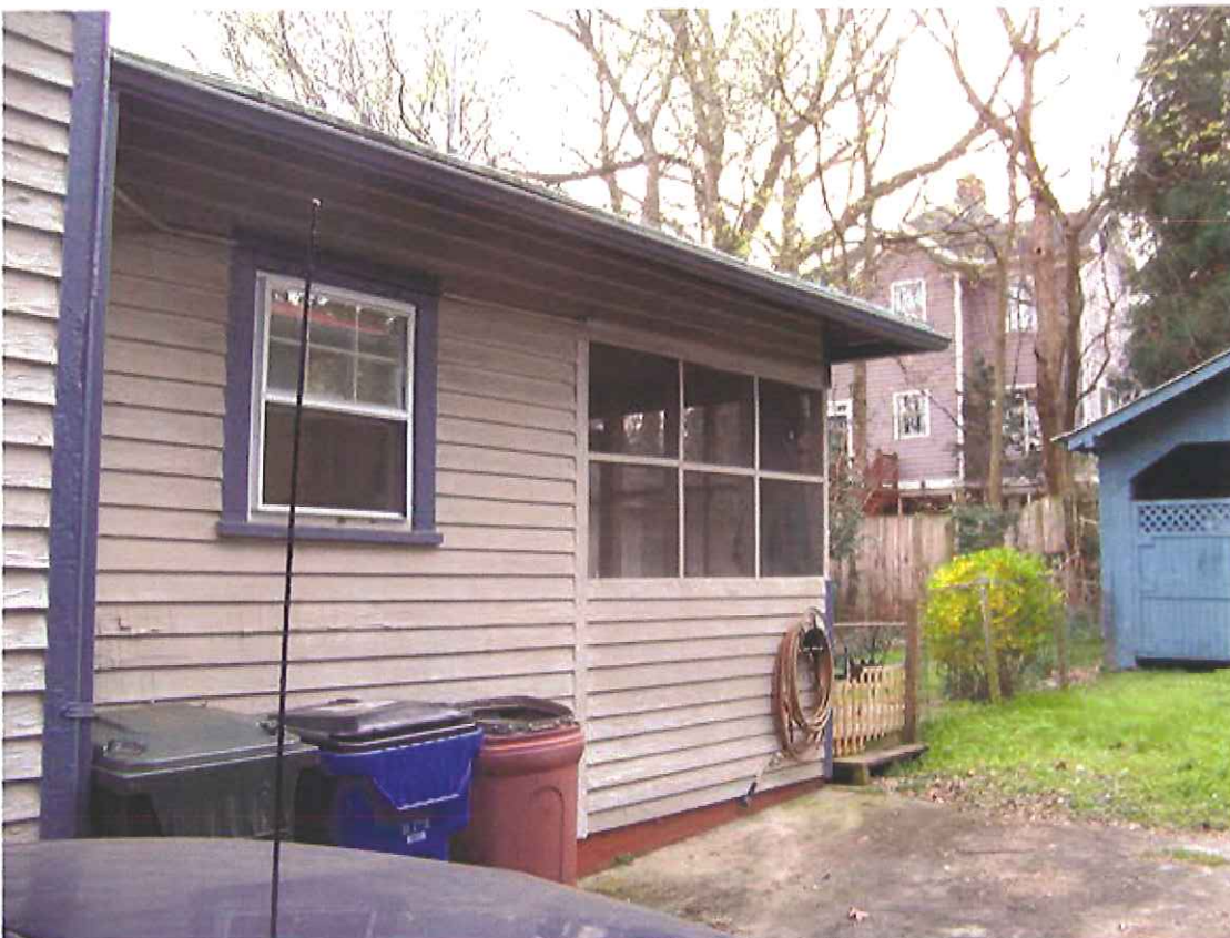
North facade, partial view showing screen porch
