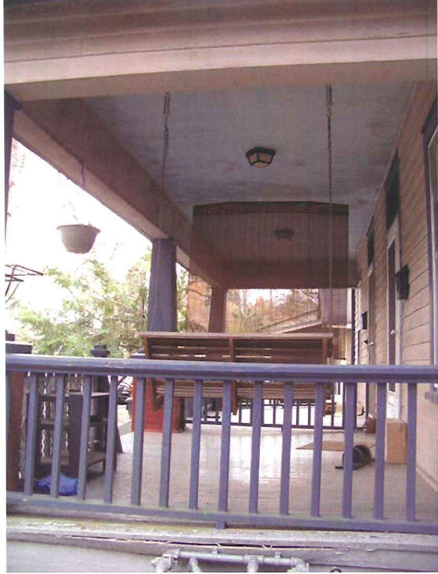
View of front porch from north side
