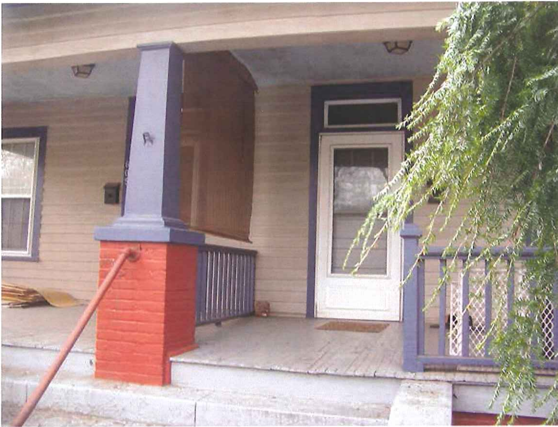
View of front porch, north side
