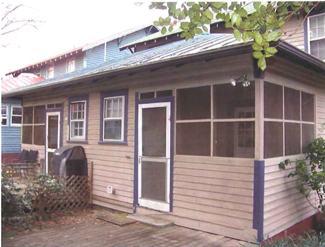
View of west facade, existing porch on southwest corner of residence
