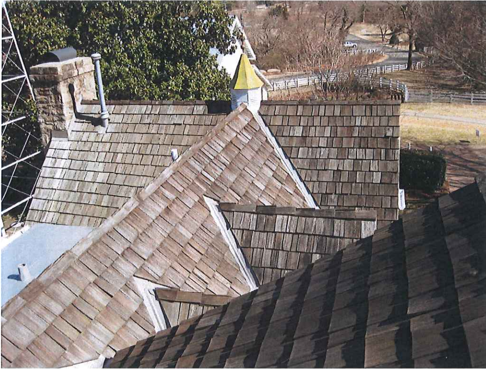
OAK VIEW MAIN HOUSE - ROOF
