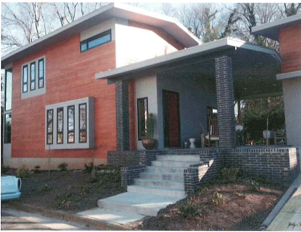
Painted front door and overall view of where screened in porch will be.
