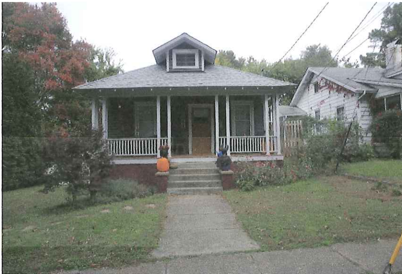
View from the street. South Elevation
