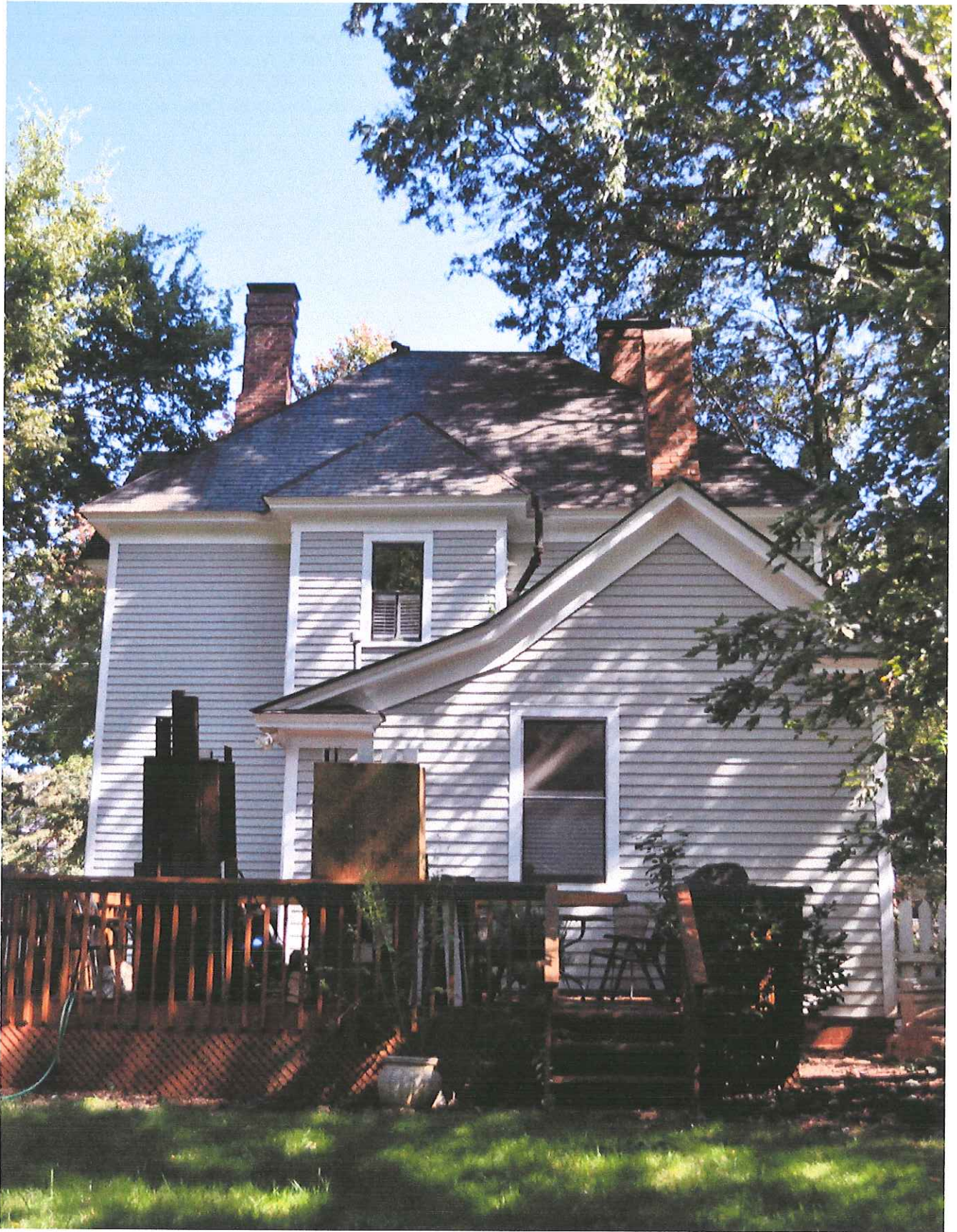
Existing Rear Elevation, interior construction debris on porch
