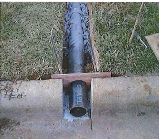
Figure 7: Cast Iron Discharge Pipe (at curb)
