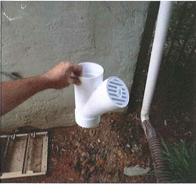
Figure 3: "Wye" Adapter for Gutter Conveyance
