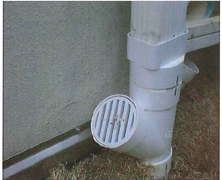
Figure 4: "Wye" Adapter and Stainless Steel Hemming Edge
