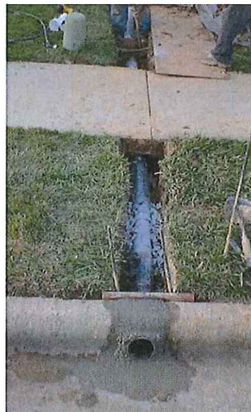
Figure 8: Cast Iron Discharge Pipe (under existing sidewalk)
