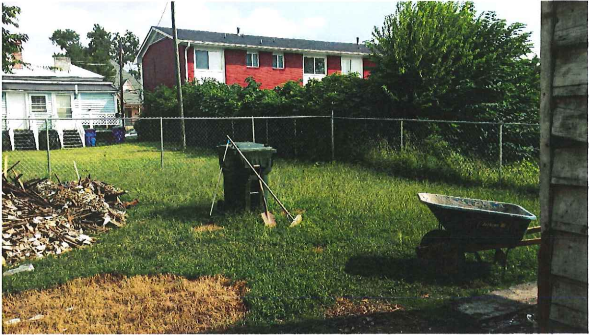
2. 222 Lenoir St – 1/1 Windows at Rear
