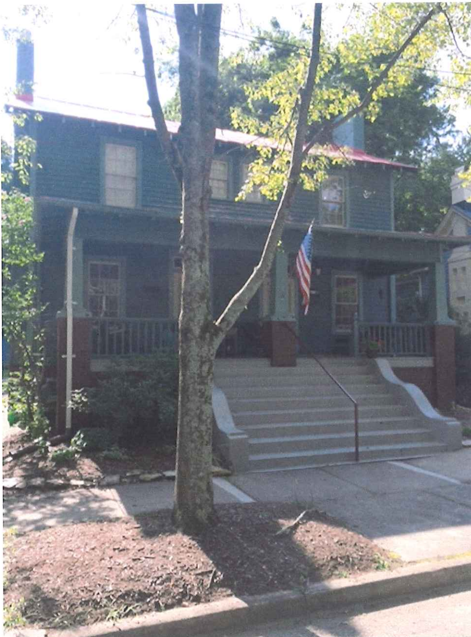
609/611 N. East Street - Front
