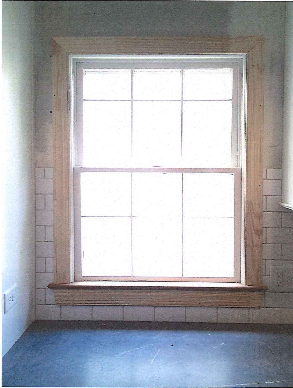
Existing window interior
