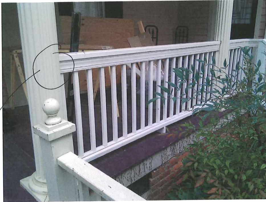
EXISTING EAST SIDE HANDRAIL (Recently added. Primo Design/Build COA)
