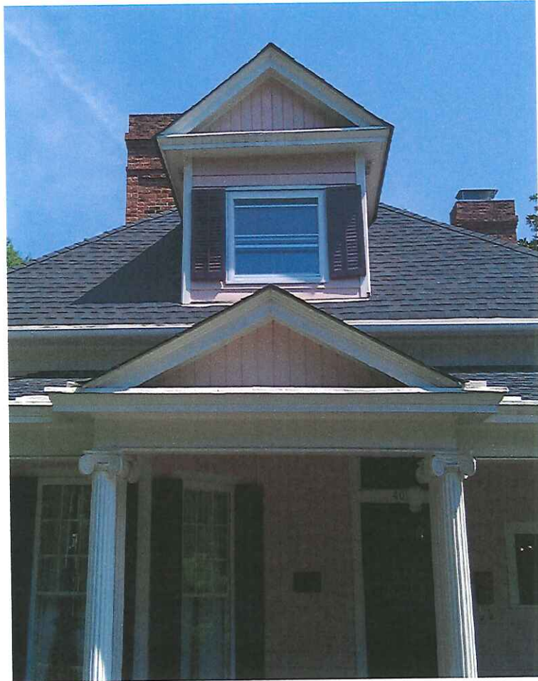
EXISTING FRONT ELEVATION VIEW
