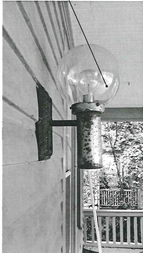
SIDE VIEW OF EXISTING LIGHT FIXTURE
