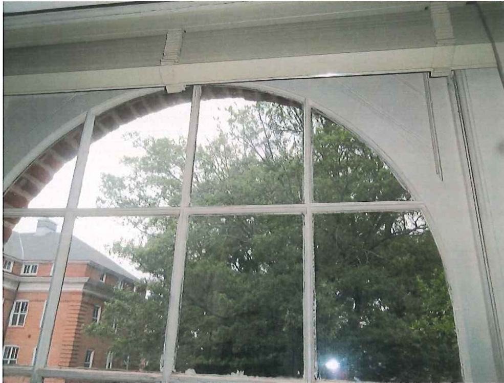
Existing condition (men's rm-104A and women's rm-204A)
