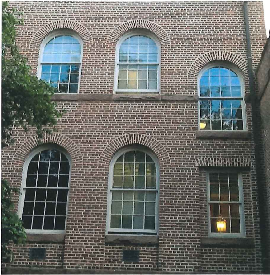
Existing exterior condition (men's and women's room)
