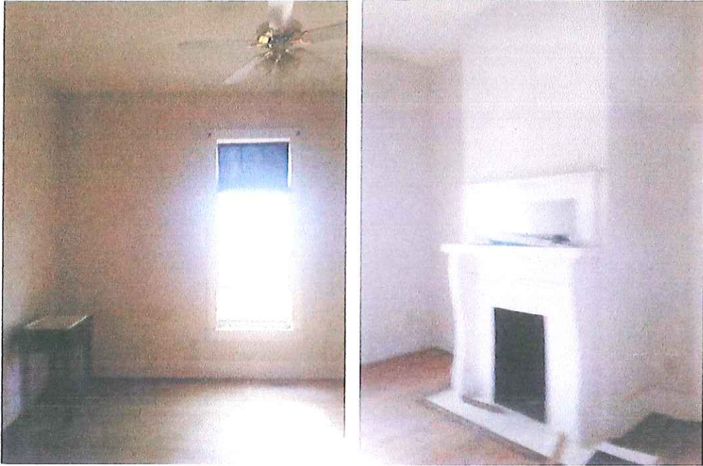
Historic Two Front Rooms dry and preserved.
