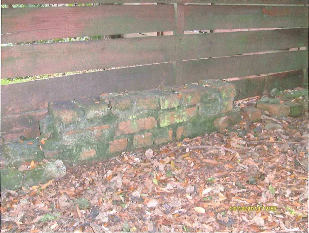
Existing wall on rear property line at 400 Kinsey St.
