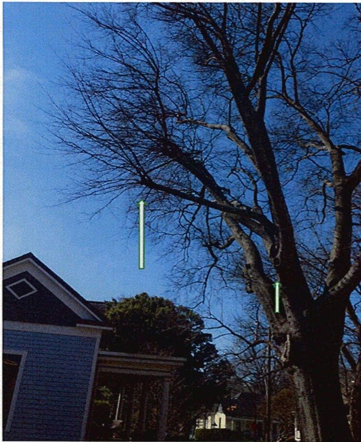
Crown that was cut back previous. Storm broken limbs . cavities in main portion of tree
