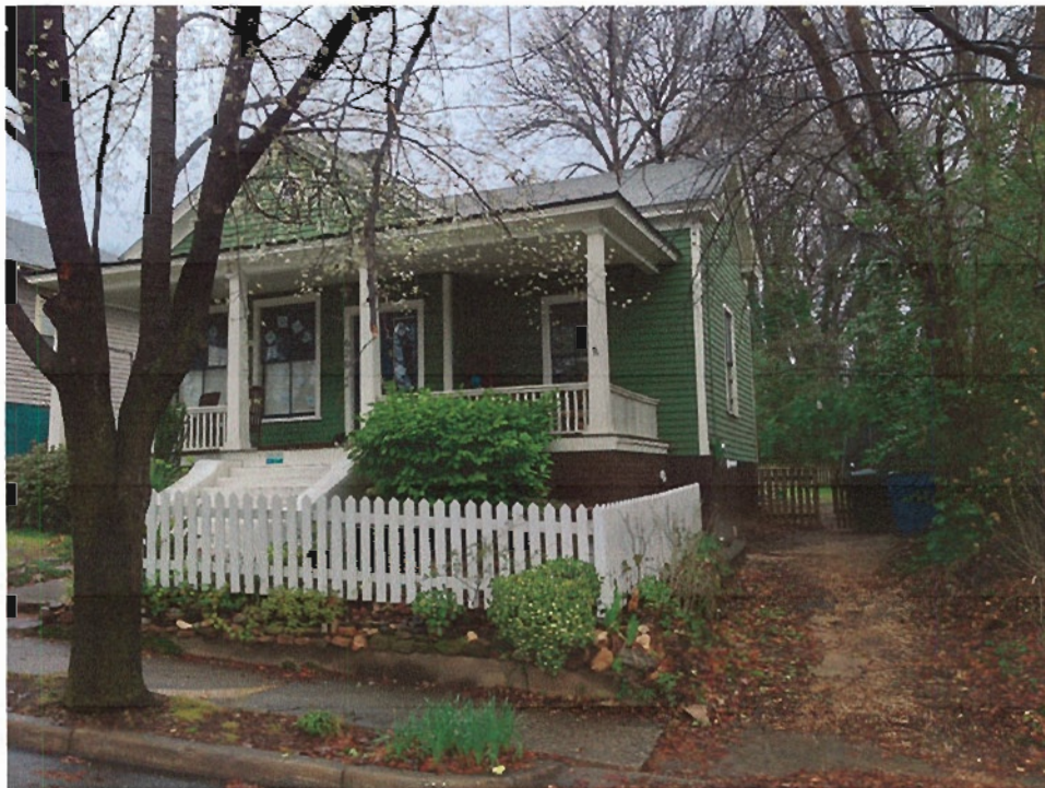
Fig 2. South elevation including view into east side yard.
