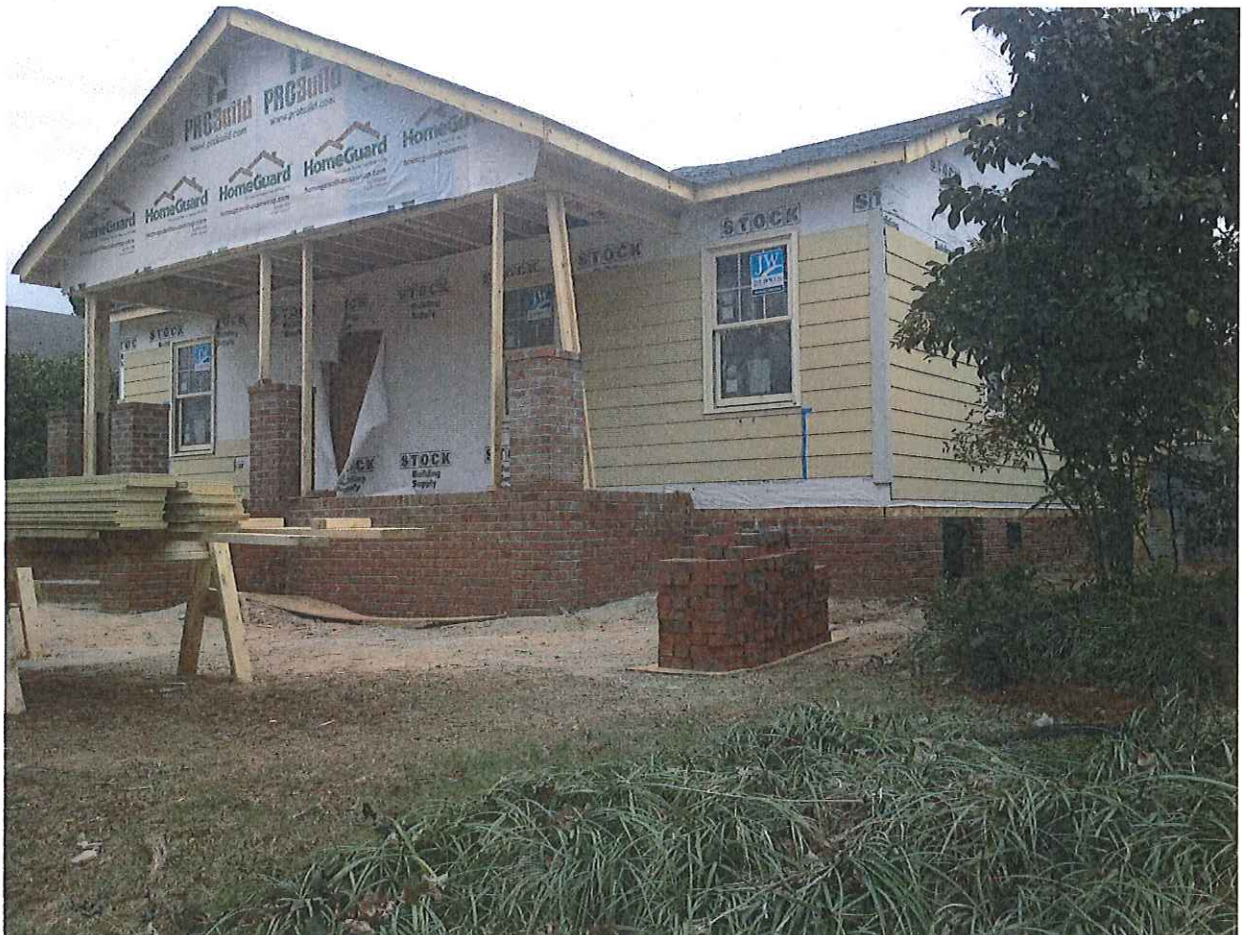
Minor Work Pic's 003
