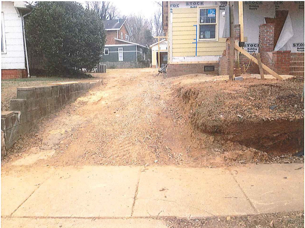
Minor Work Pic's 005
