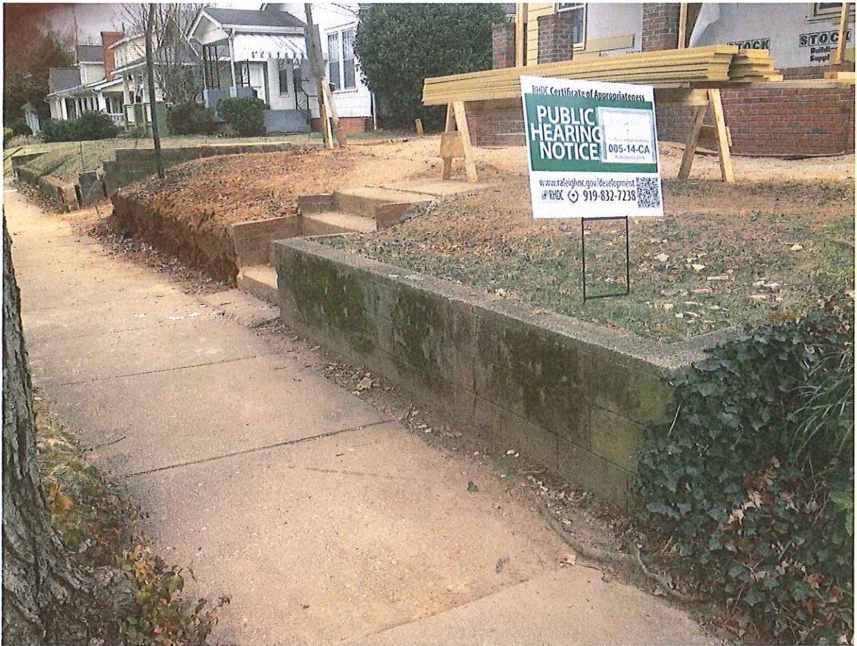
Minor Work Pic's 004
