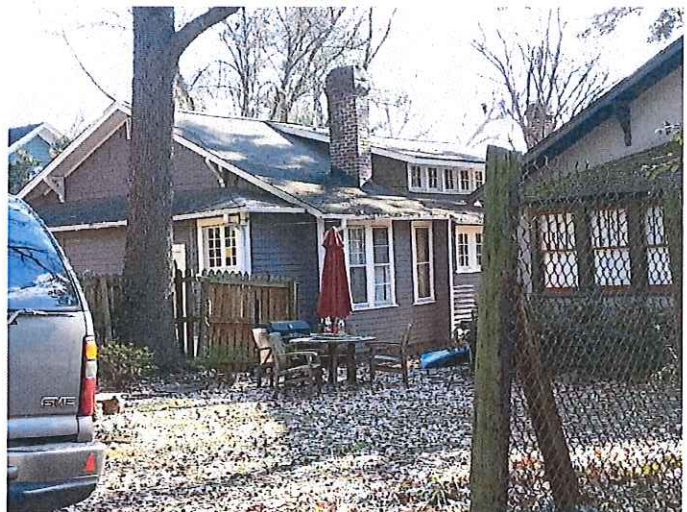
Rear view of chimney and kitchen windows to be altered
