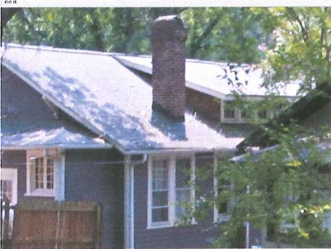
Existing taken from neighbors back yard
