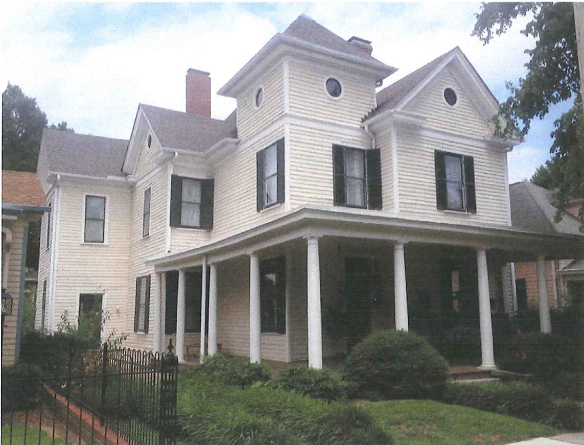
405 Polk Street Front facade
