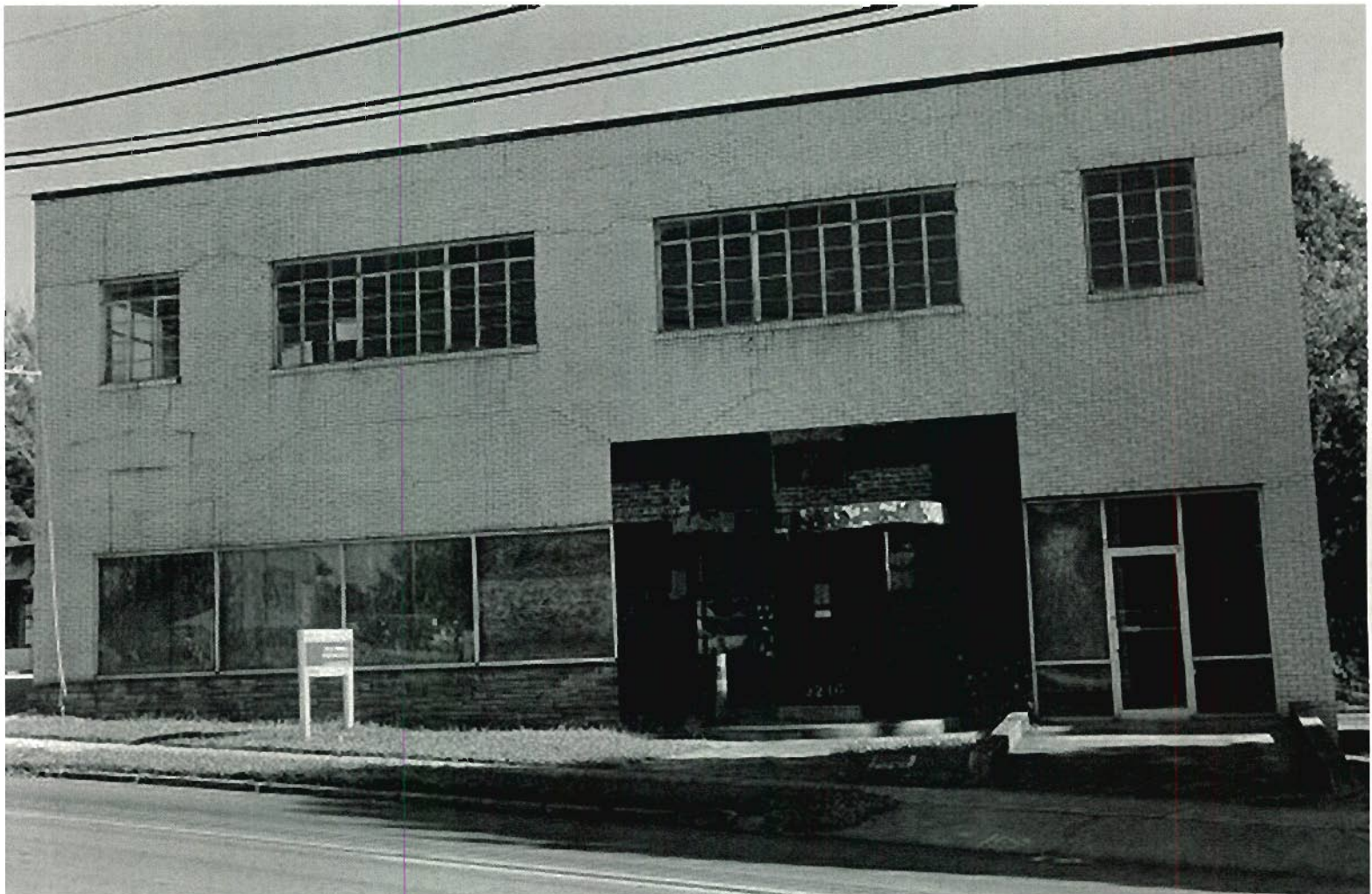
Existing front (South) facade
