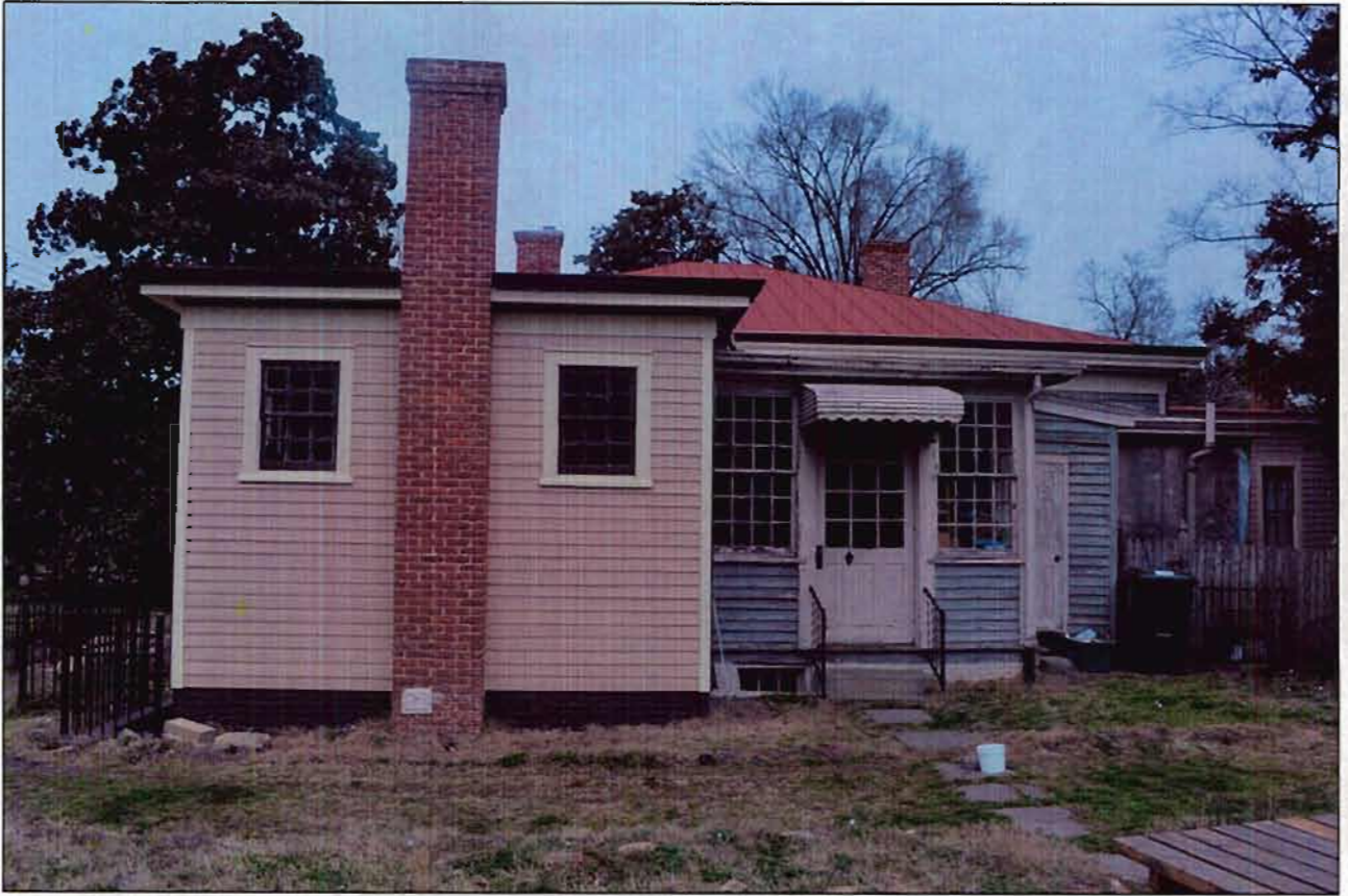
South side of house
