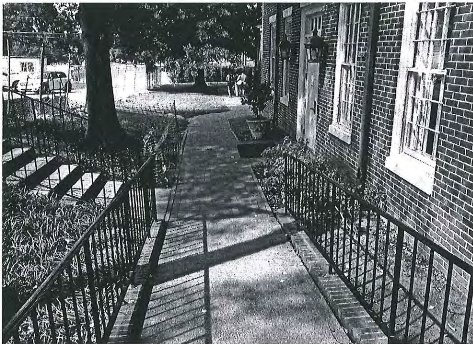
Photo 7. Existing walkway to be replaced. Belk Dining Hall west side dining room entry door right, new Book Store west or left in photo. Note existing mature tree (note 1 in photo, left of walkway) shall be protected and maintained.
