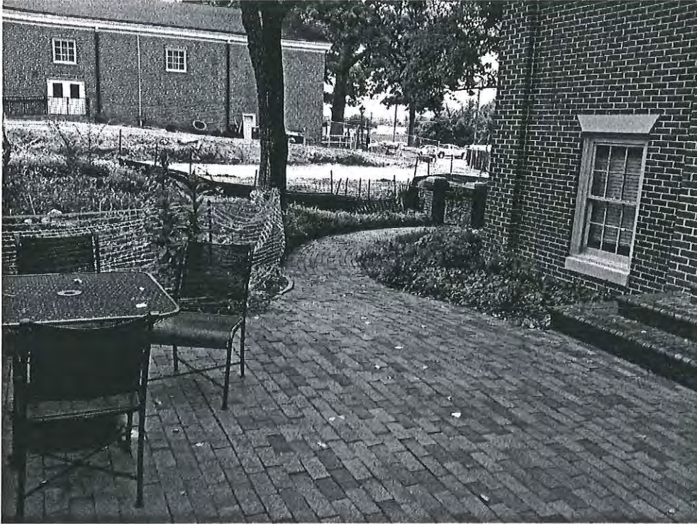
Photo 10. Existing window on west elevation of Belk to be removed and replaced with door. Note existing landscaping in this area shall be removed and grade dropped to create an entrance to elevator lobby at the lower right window opening. Photo is taken standing on existing walkway.
