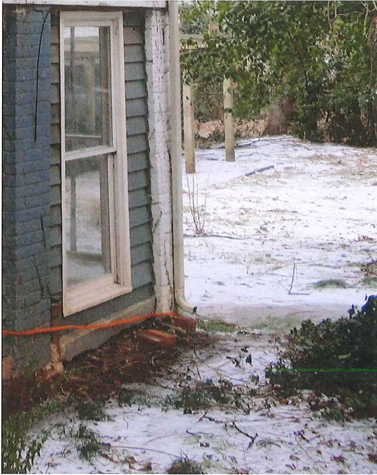
Exterior North side of house – screen porch window
