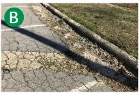
Buckled and cracked asphalt in parking lot
