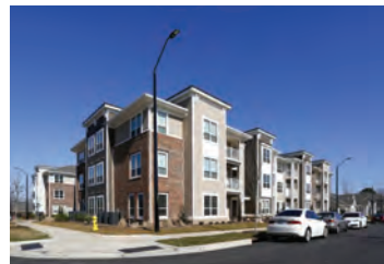
THREE-STORY SUBSIDIZED RENTAL HOUSING The Village at Washington Terrace, Raleigh, NC
